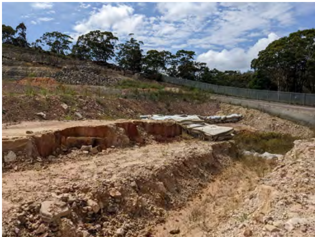
Site south – South cell facing east, stormwater diversion using mattresses.
